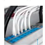
Inner wall beneath floor: Roxtec ComSeal™ around power cables for optimized cooling and energy saving.
