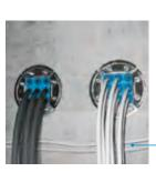
**Foundation:** sealing of power and control system cables going through core drilled holes.
