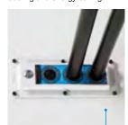
Cabinet structure penetrations: Roxtec CF 16 for signal cables coming up to the servers.
