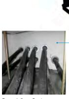
**Beneath floor:** Single power cables sealed air tight with Roxtec round seals.
